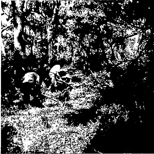
Trail construction Dharug National Park
