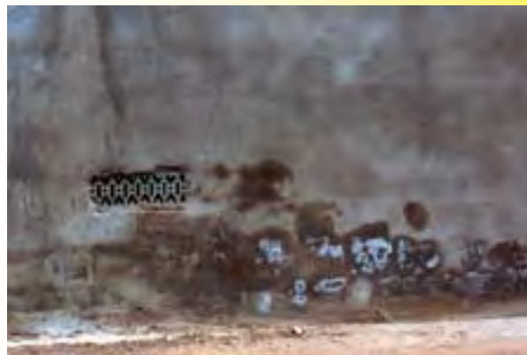
Render showing signs that excess salt and water are present Photo: NSW Agriculture
