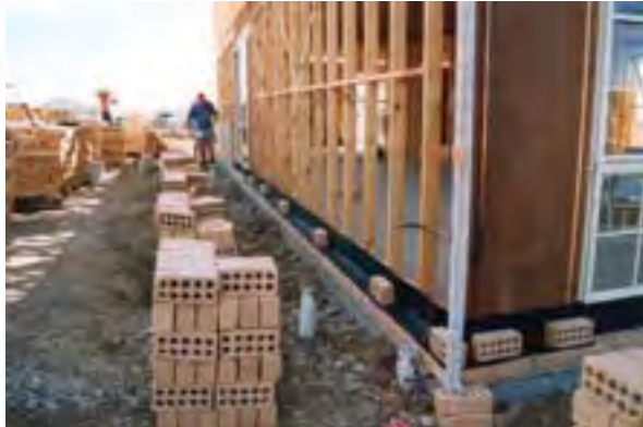
Installation of polyethylene sheeting in mortar joint of the brick work - Photo: DIPNR
