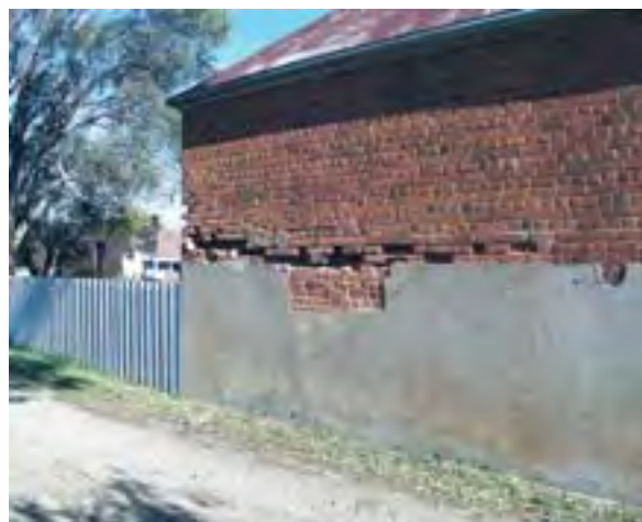
A non permeable render has decreased evaporation Photo: NSW Agriculture
