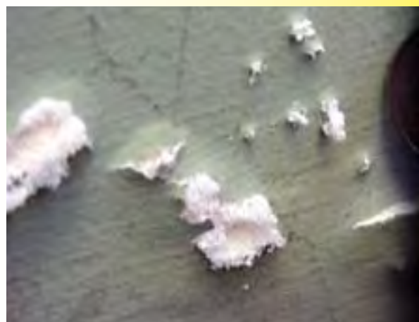
Paintwork blistering due to the accumulation of salt Photo: DIPNR
