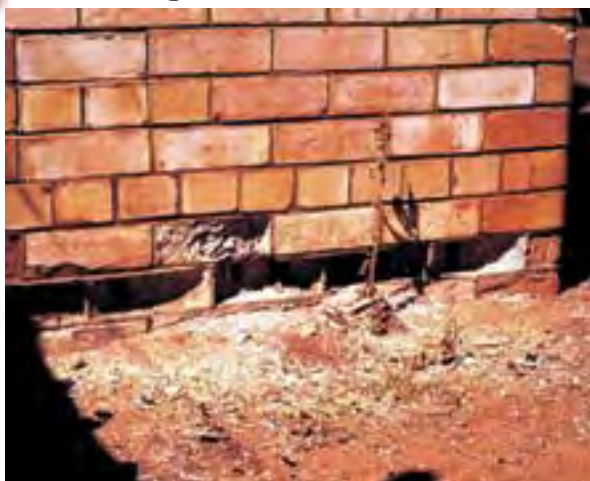
Brick work showing the effects of fretting Photo: NSW Agriculture
