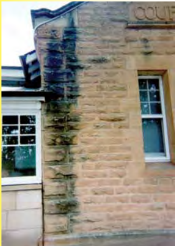
Courthouse showing symptoms of falling damp from a blocked gutter - Photo: NSW Agriculture
