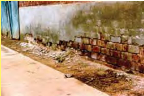
Damp-proof course has been bypassed by rendering Photo: NSW Agriculture
