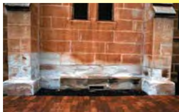
Sandstone showing signs of salt and water damage Photo: NSW Agriculture
