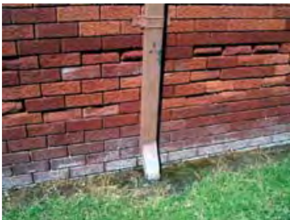
Rusted down pipe allowing rainwater to mobilise salts in the soil. - Photo: DIPNR
