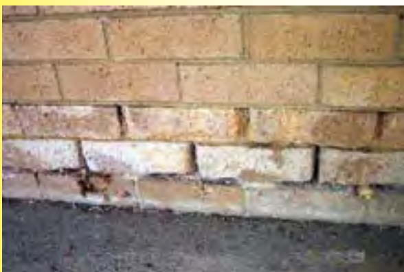
Damp-proof course limiting damage to lower three bricks Photo: DIPNR
