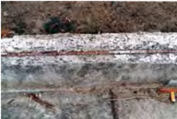
Reinforcing steel exposed and corroding Photo: DIPNR
