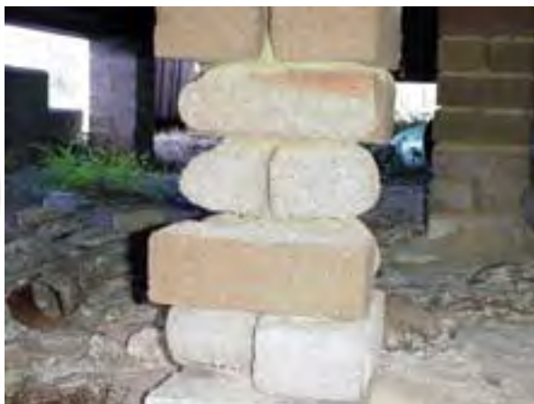
Bricks exhibiting signs of salt and water damage Photo: DIPNR
