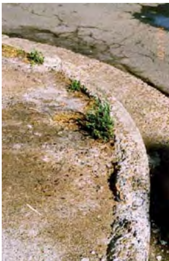
Kerb and guttering affected by sulphates Photo: DIPNR
