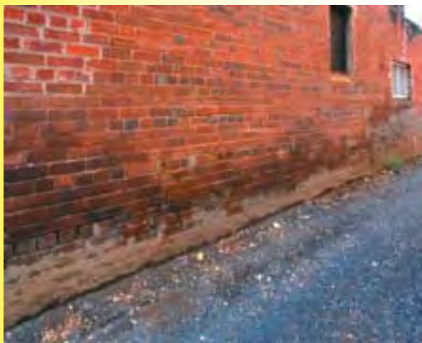
Building with wet 'tide' mark - Photo: NSW Agriculture
