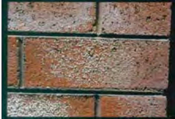
Bricks efflorescing - Photo: NSW Agriculture
