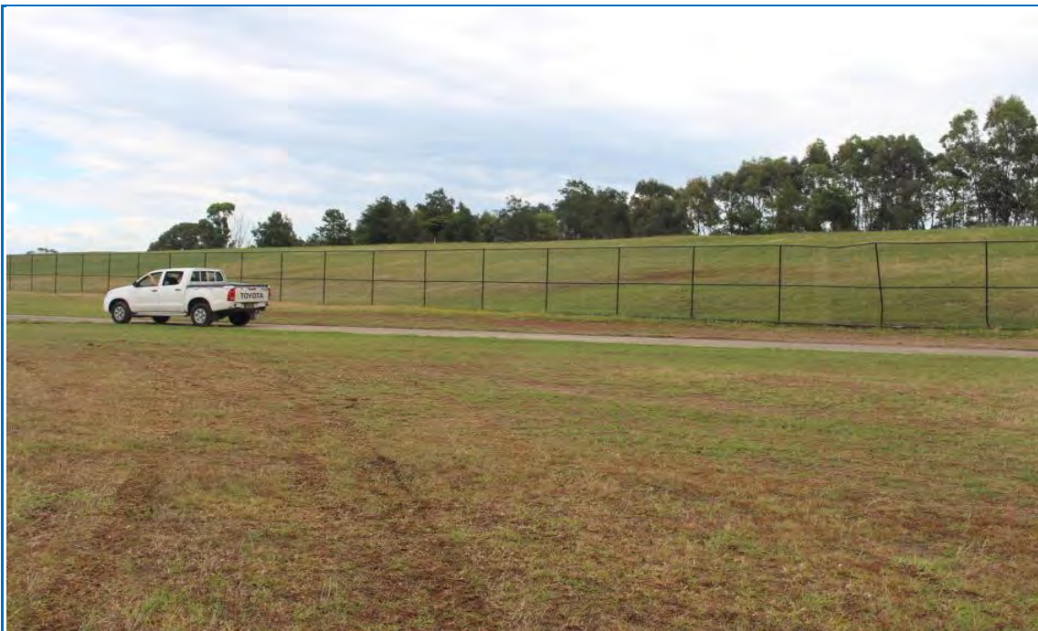
Figure 4.4: The earth wall in the background has been constructed from materials taken from the foreground in this image and other areas within the fenced PCC building complex
