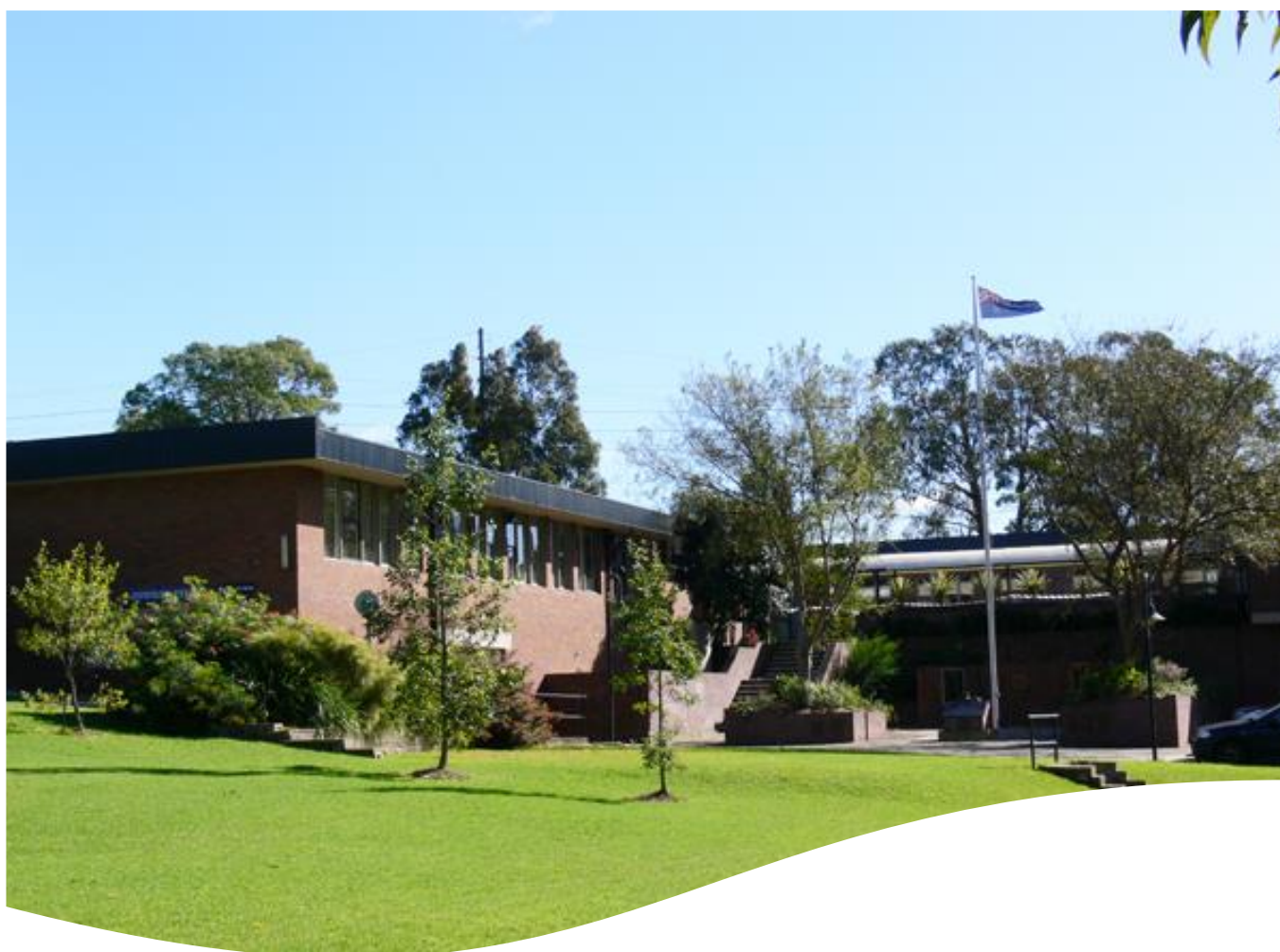
Image 16. CSNSW Academy Administration Building
