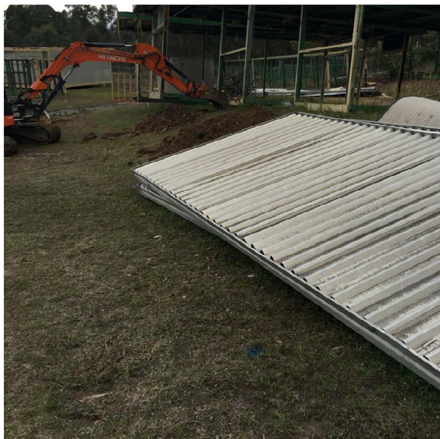
Photograph 12 - Looking south west over SP8
