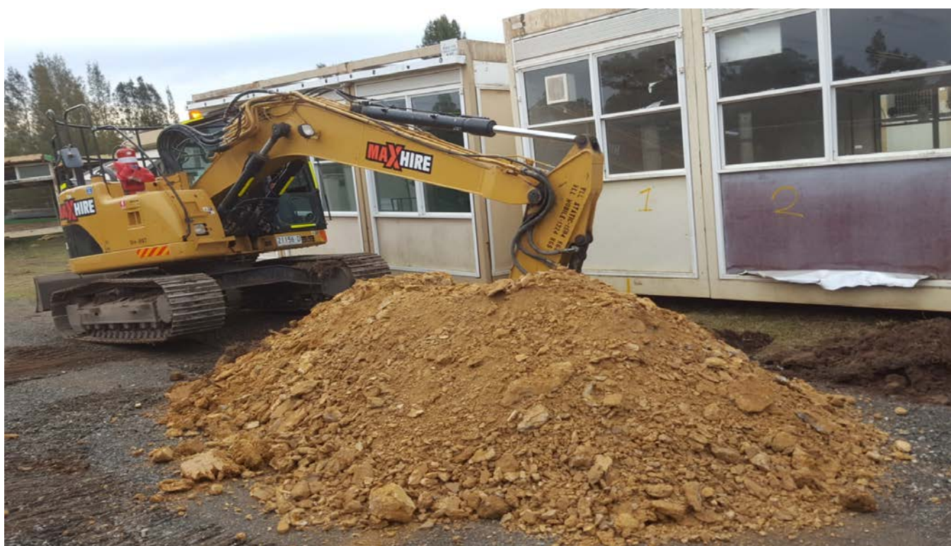
Photograph 18 - Orange residual soils/ weathered rock excavated from below overlying topsoil/fill
