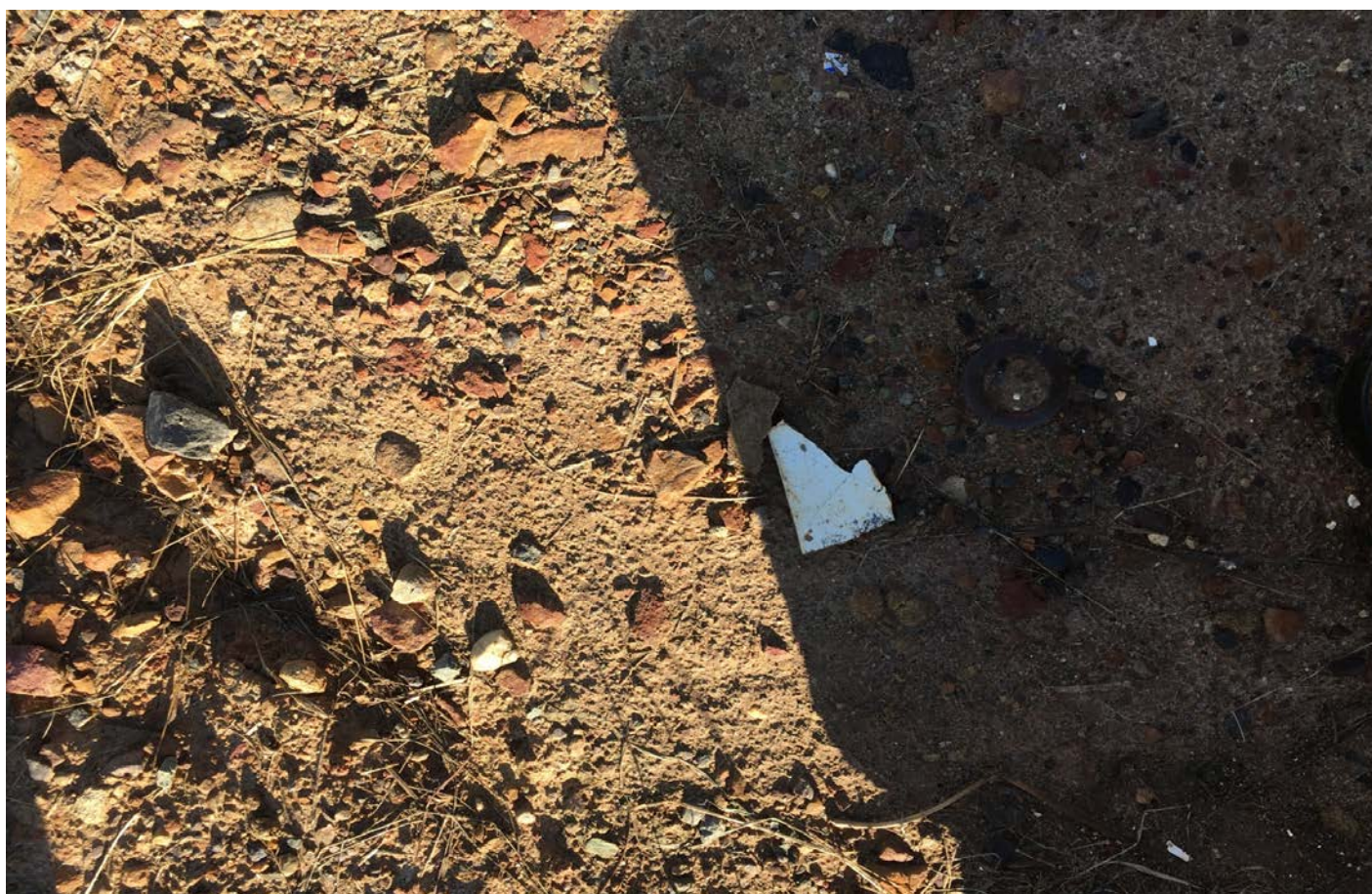
Photograph 4 - Potential ACM from demountable eves (ACM 3)
