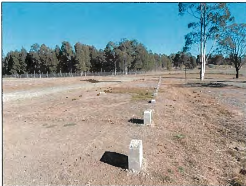
Figure 9: Area 2 – Demountable building piers and filling terraces
