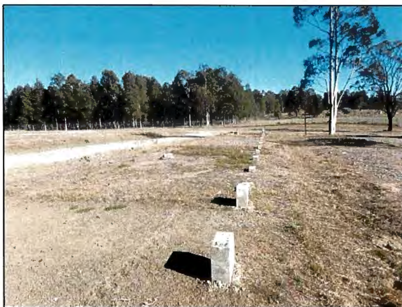
Figure 5: Area 2 – Demountable building piers and filling terraces
